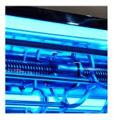
Ultraviolet C (UV-C) technology has been a popular method for preventing the accumulation of airborne pathogens on HVAC equipment for many years now. UV-C bulbs
